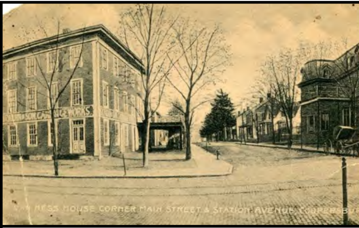
Vintage photo of S. Y. Kern and Son Carriage Works.
