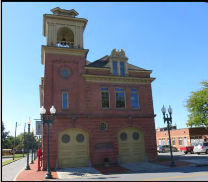
The Pennsylvania National Fire Museum in Harrisburg, PA
